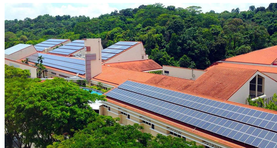
Singapore American School, 1.2 MWp
