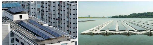
HDB Rooftop Solar PV Floating Solar PV
