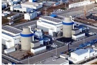
Haiyang- China AP1000 In Operation
