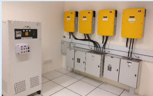
Transformer & inverters
