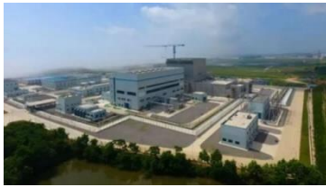
HTR-PM, China 2x110 MWe HTGR In Operation
