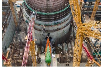
Rooppur 1&2- Bangladesh VVER-1200 Under Construction
