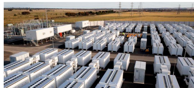
Victorian Big Battery: Virtual Transmission Line, 250MW SIPS 300MW/450MWh
