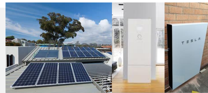
Dist. BESS/Virtual Power Plants: Islanding, contingency FCAS & dispatch ~700MW/1900MWh
