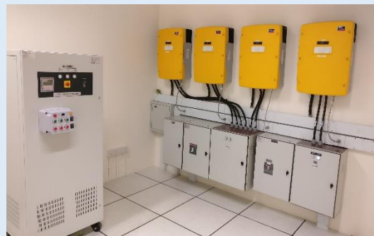
Transformer & inverters
